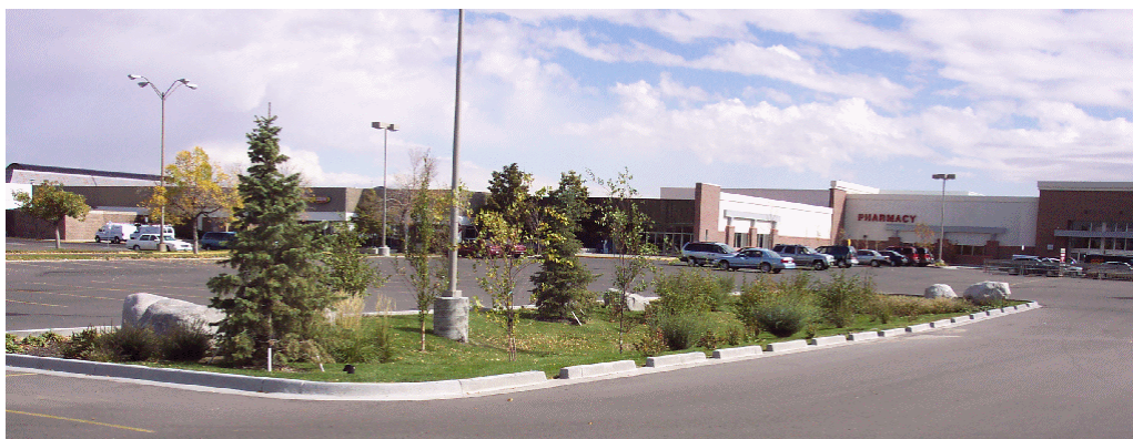
Porous landscape detention in an Aurora parking lot. (Photo Courtesy of Michelle Delaria, CASFM photo database, http://www.casfm.org/stormwater_committee/ )
